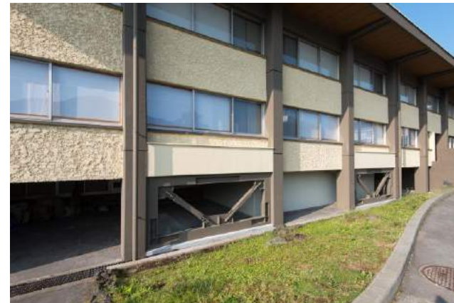
Seismic Retrofitting selesai
