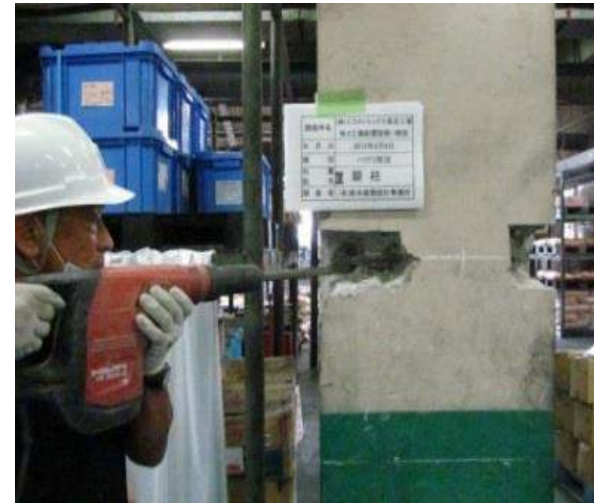
Sample coring diuji kuat tekan
