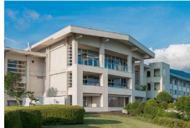
Seismic Retrofitting selesai
